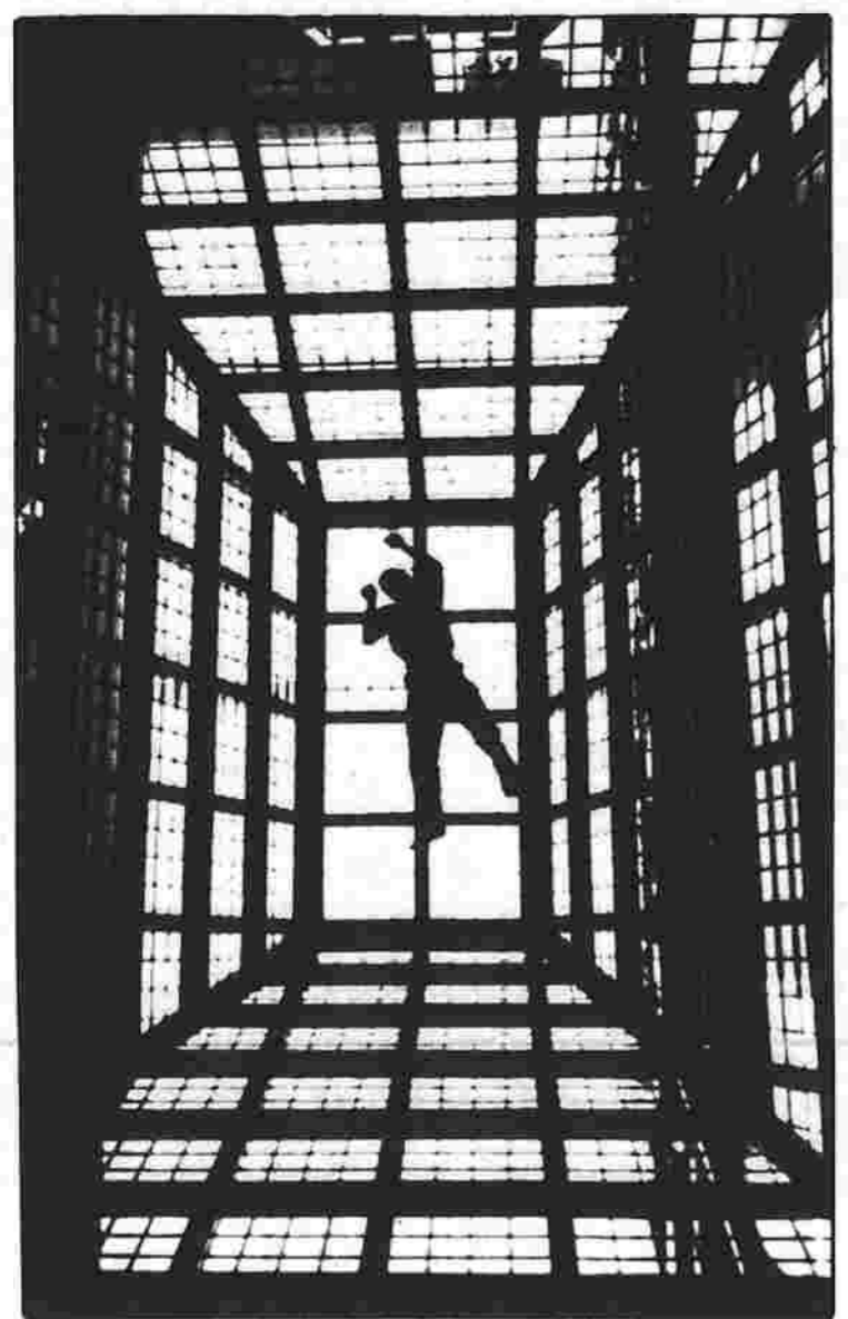
Utility engineer Greg Jones checks the grill work of the 25-foot canopy above the meeting rooms at the Cincinnati Hotel in Cincinnati. The hotel, which was constructed in 1882 as the Palace Hotel, reopened in February after a $23 million renovation that took two years.
